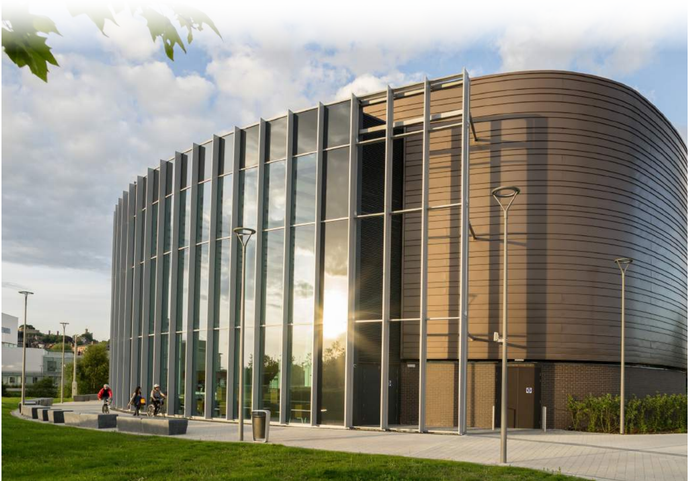
The curved building facade features bronze rainscreen cladding
